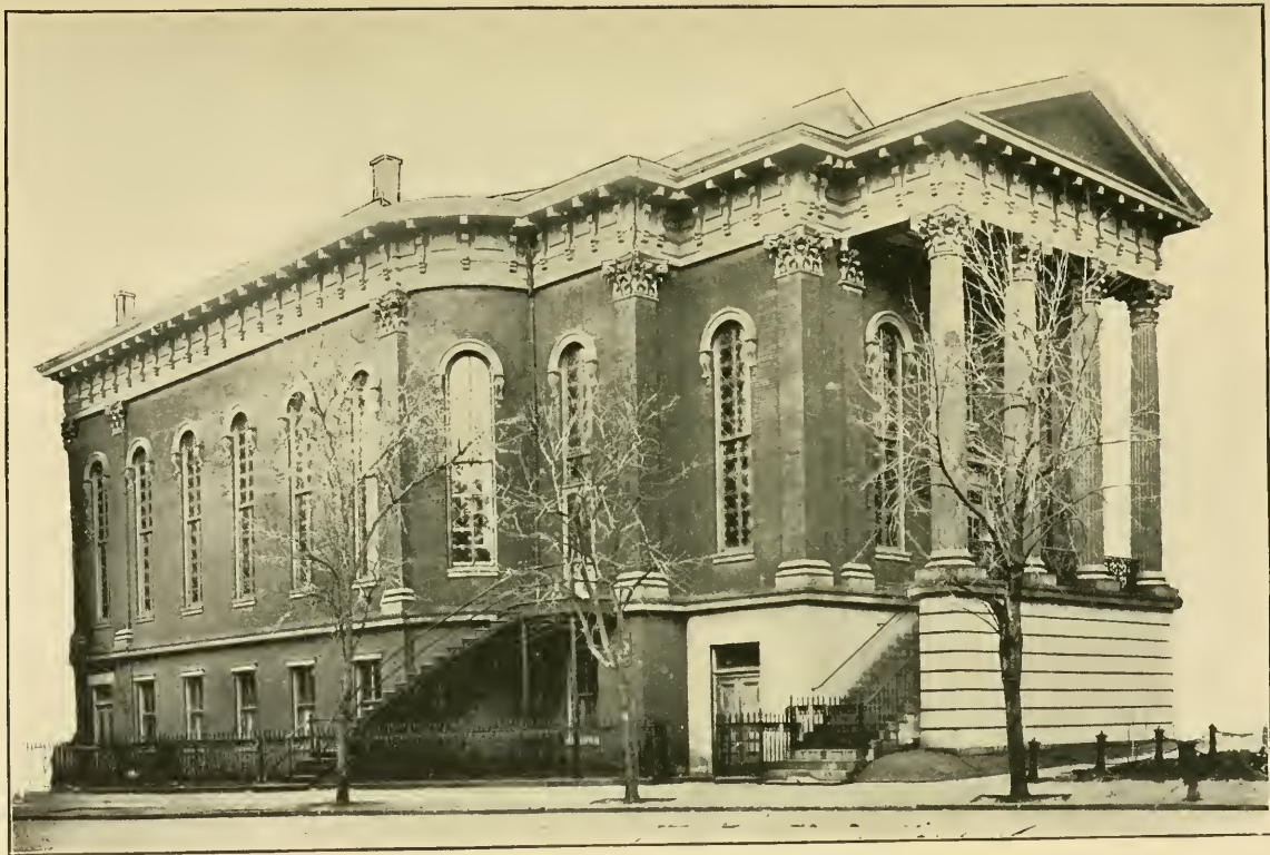
THE NEW YORK AVENUE PRESBYTERIAN CHURCH.
